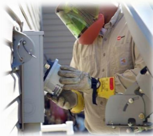
AMI Meters 894,000 Additional Meters
